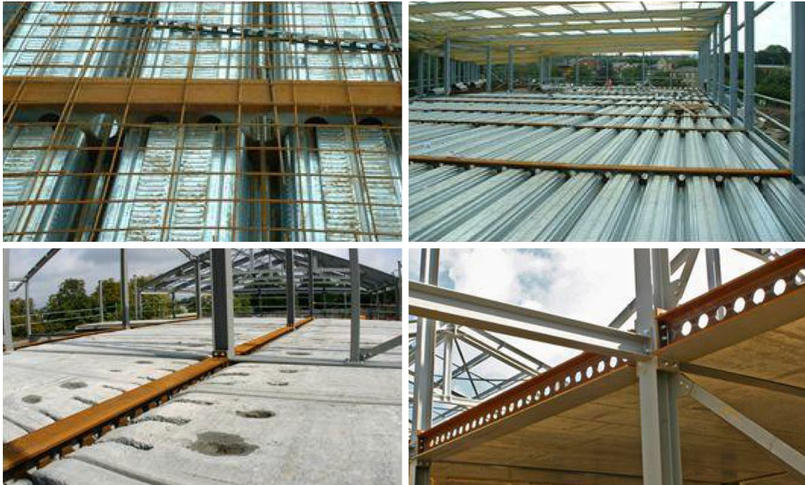
Figure 2. USFB ® used with profiled steel decking (top) and with the precast concrete unit (bottom) (Tsavdaridis et al., 2013).
